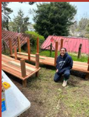
FSL student helping in the construction of the raised beds
